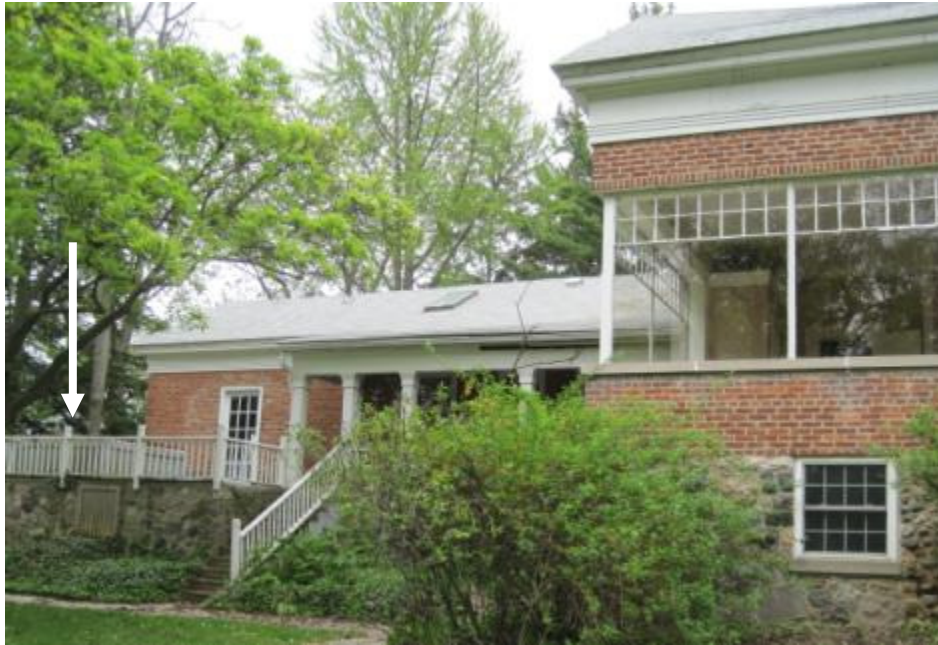
Looking west at rear of house, arrow indicates existing hot tub, May 2011
