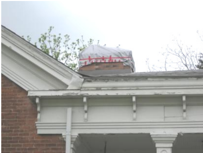
Detail of chimney proposed for removal, looking south, May 2011
