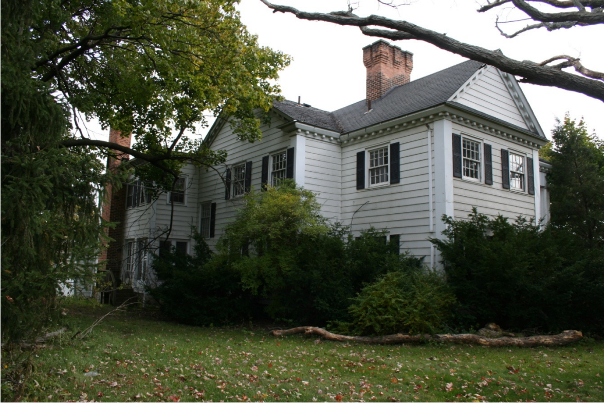
North and west elevations looking southeast, October, 2009
