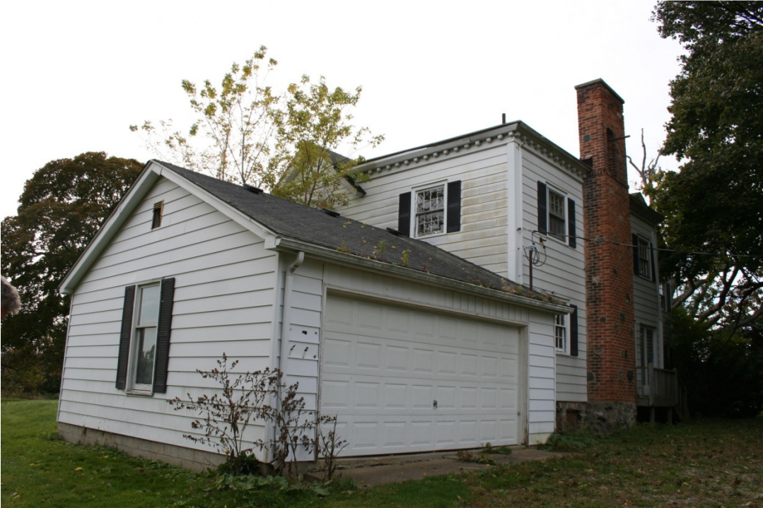
East elevation looking southwest, October, 2009
