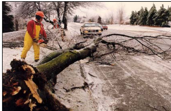
Storm Damage Cleanup
