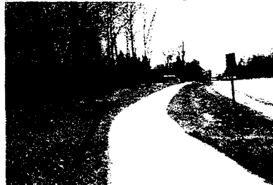
View of stormwater drainage ditch along the west border, at Livernois. This ditch empties into existing storm sewer.
