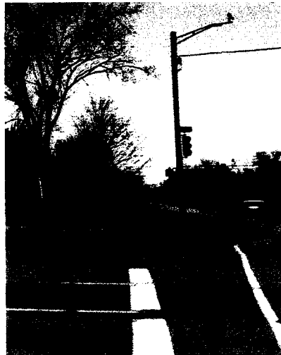
Crosswalks are provided at intersections, as well as paved paths at Livernois and Hamlin.
