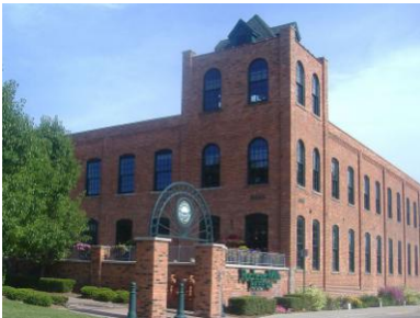
Historic Rochester Mills Beer Co., just north of the proposed theater site.
