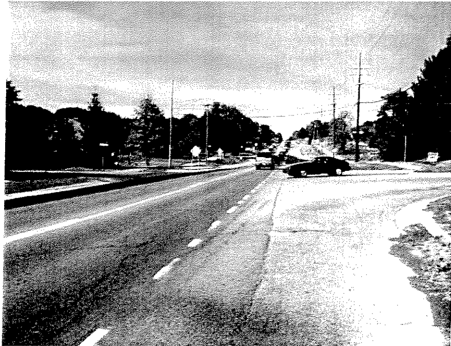
Photograph 4 - Looking westbound Tienken Rd east of Kings Cove
