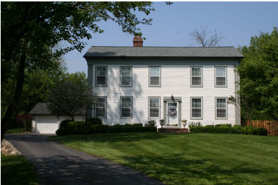
Figure 3 - 1207 Livernois, front facade, May, 2007
