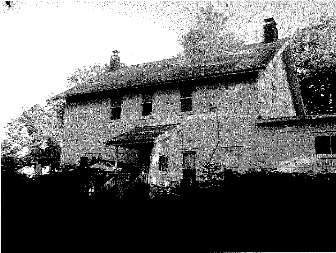
Figure 3 - View of rear from northwest. J. Dzurman, 2006.
