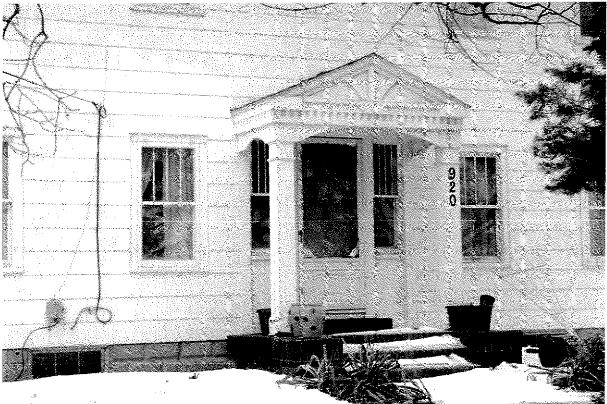
Figure 6 - Detail of front porch, K. Kidorf, February, 2007.
