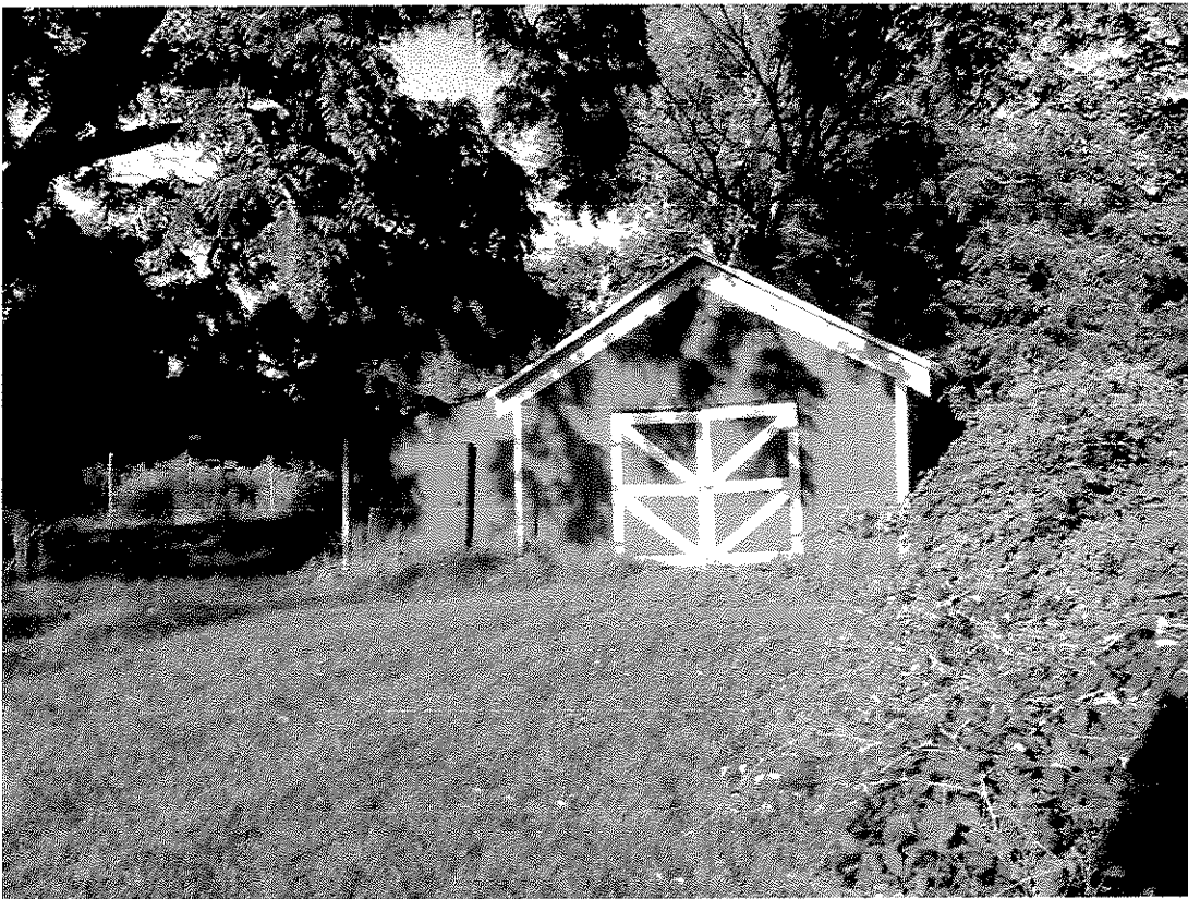
Figure 4 - View of shed from west, J. Dzurman, 2006
