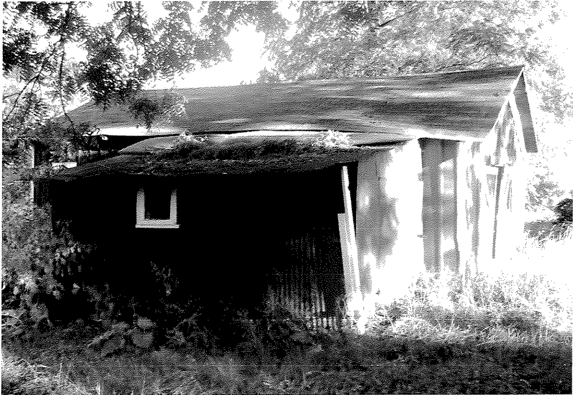
Figure 5 - View of shed from north, J. Dzuirman, 2006.
