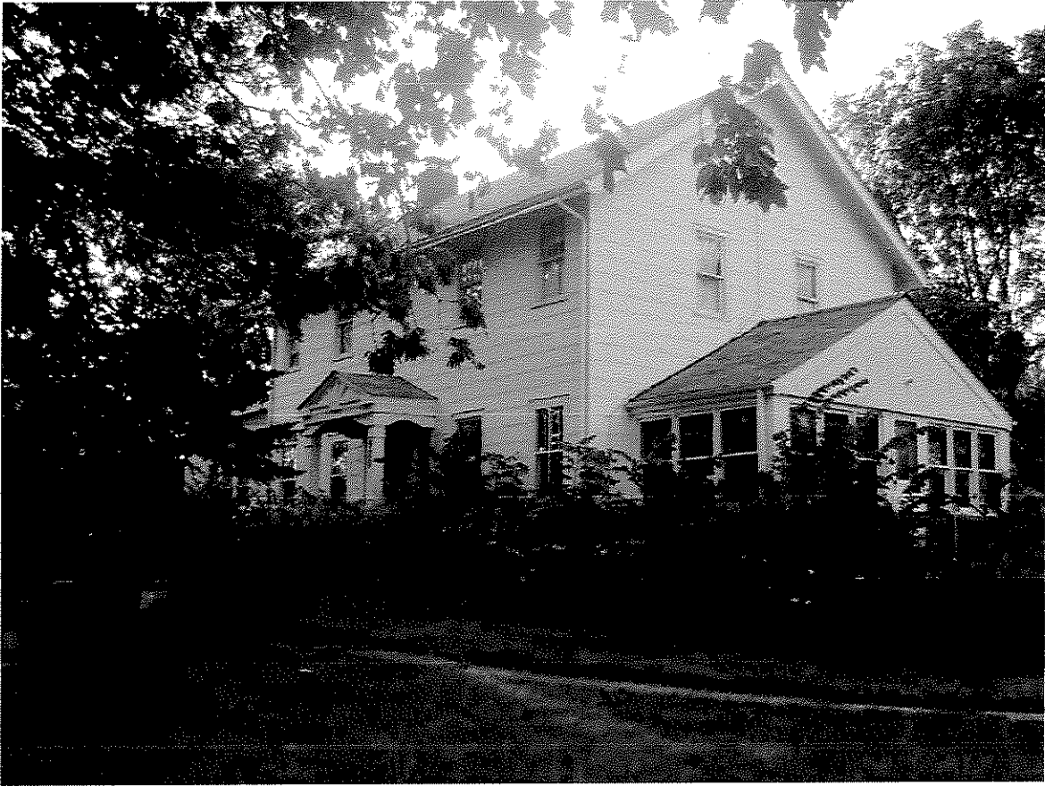
Figure 1 - View of front from southeast. J. Dzurman, 2006.
