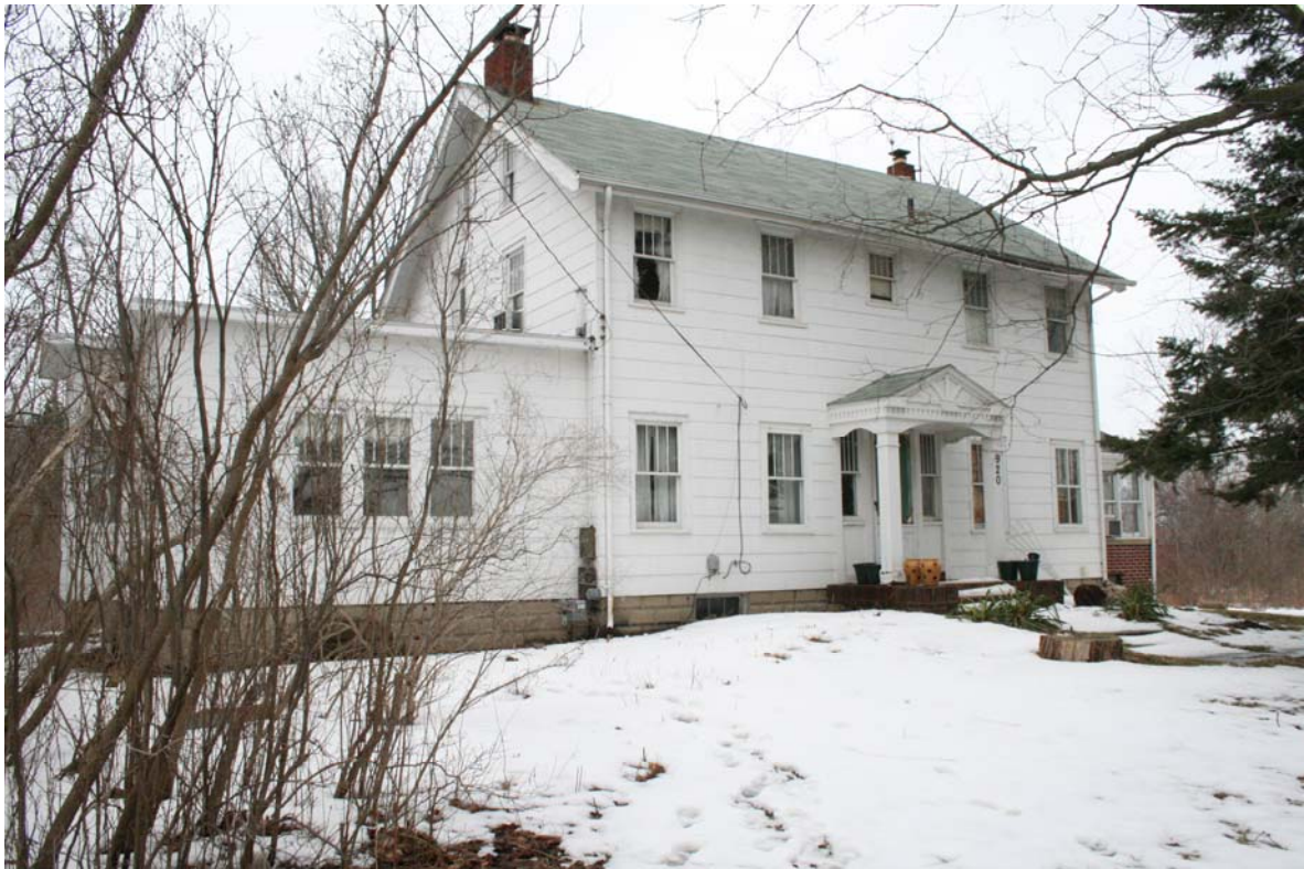
Figure 2 - View from southwest. K. Kidorf, February, 2007.
