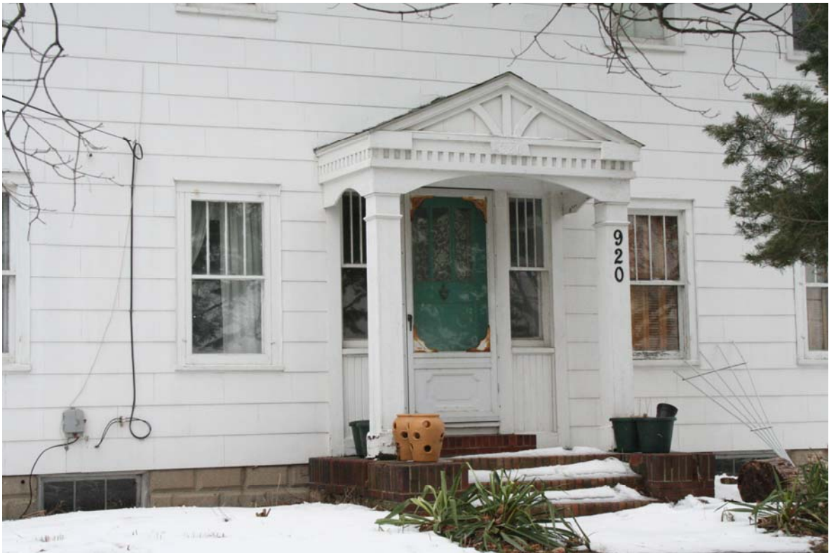
Figure 6 - Detail of front porch, K. Kidorf, February, 2007.
