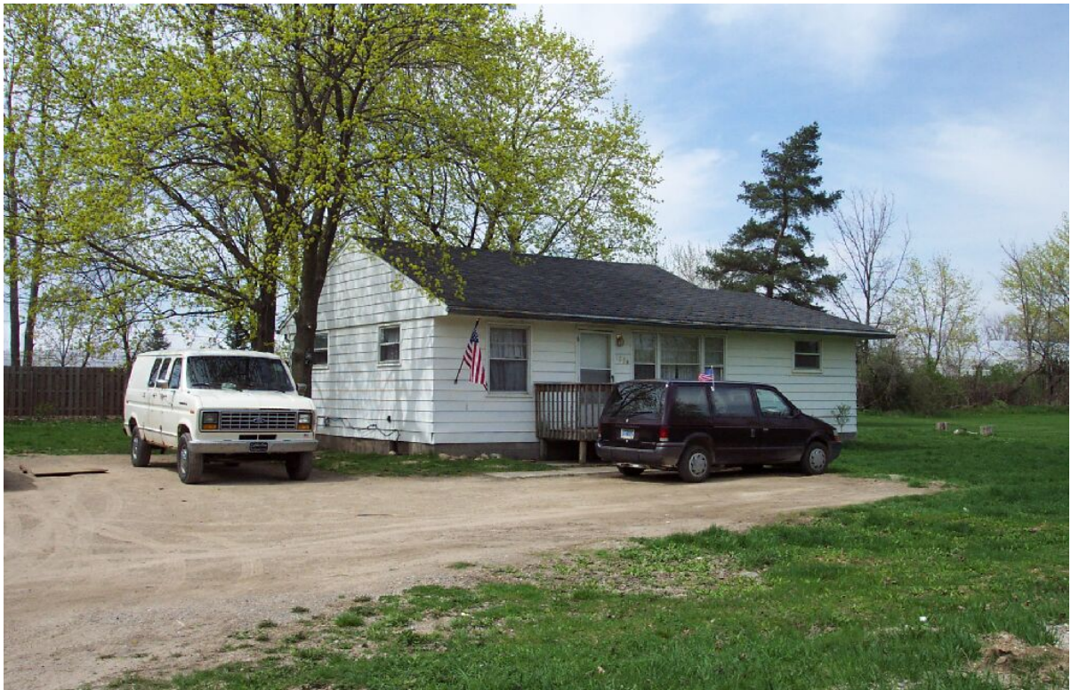
Photo 8: Ranch house at 1894 Wayside Park
