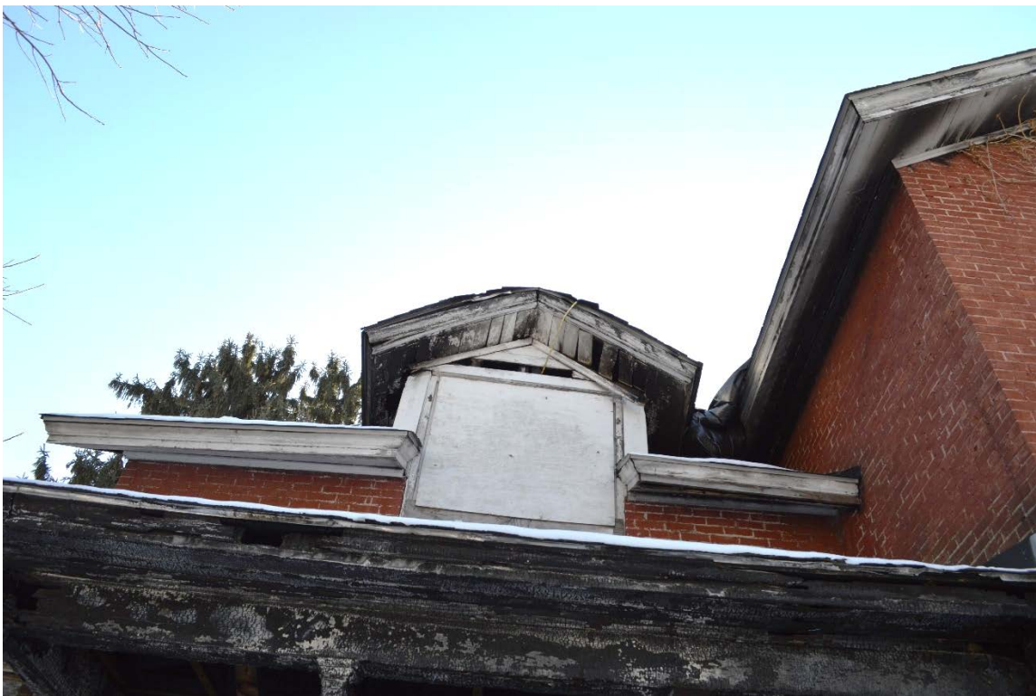
16 – North dormer showing fire damage, January 2021
