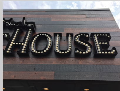
example of exposed bulb channel letters
