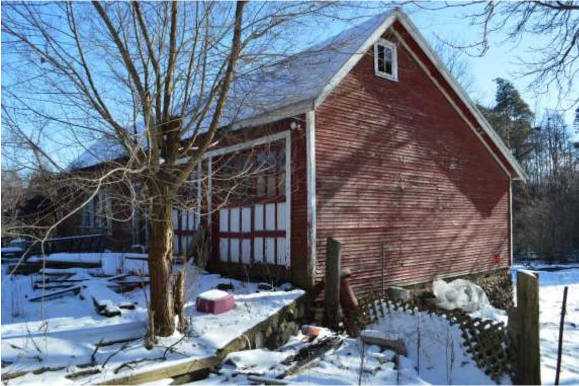
10-Looking southeast at north and west elevations of barn, January 2021
