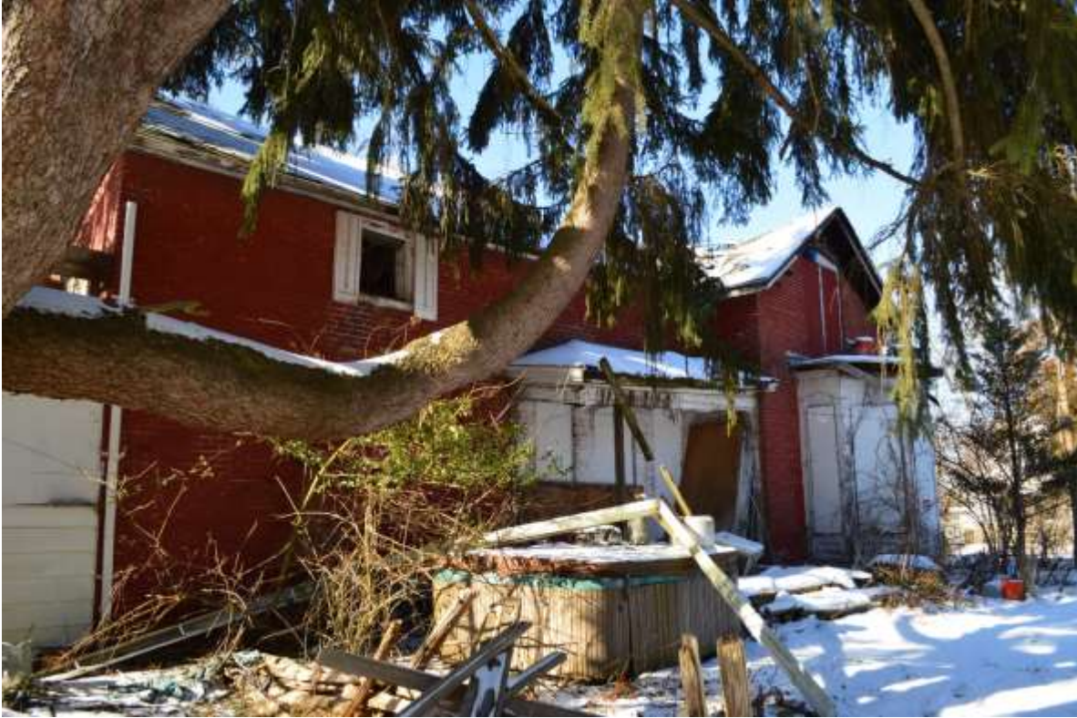
3-Looking northwest at east side of house, January 2021
