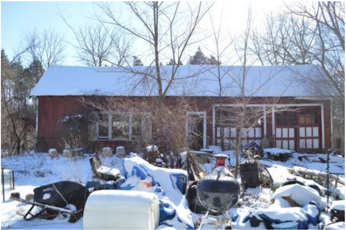
8-Looking south at north elevation of barn, January 2021
