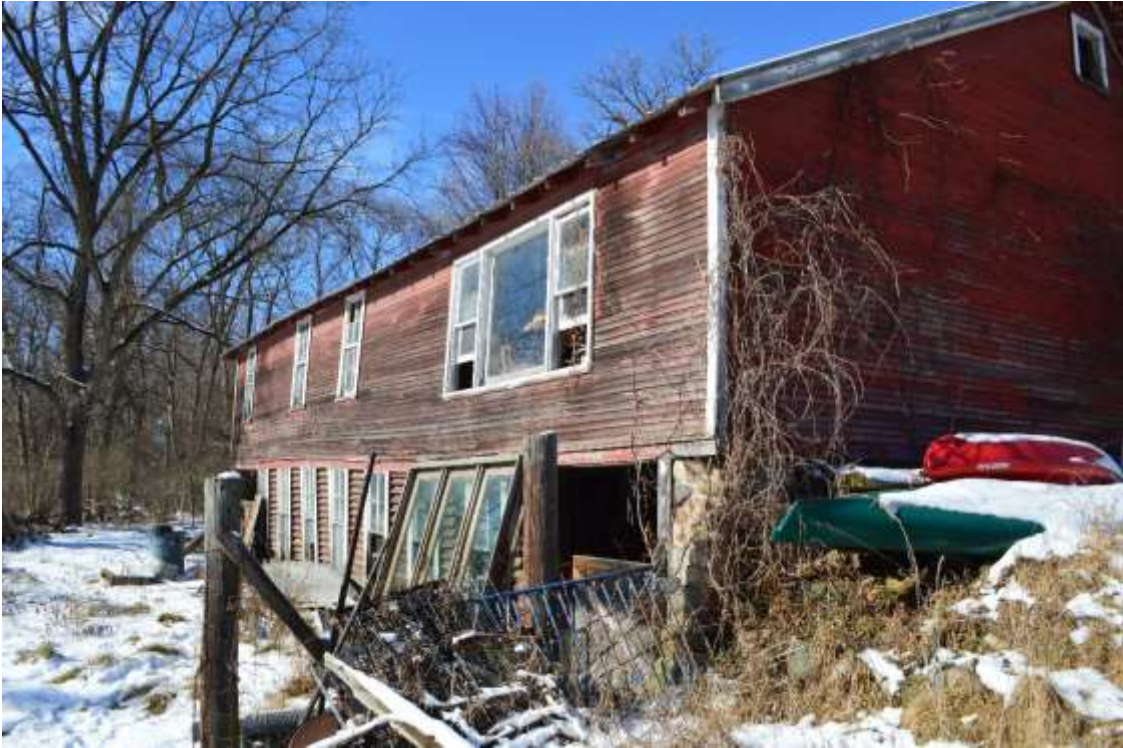
9-Looking northwest at south elevation of barn, January 2021
