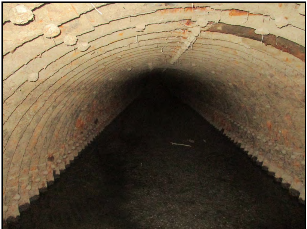
View through culvert facing north
