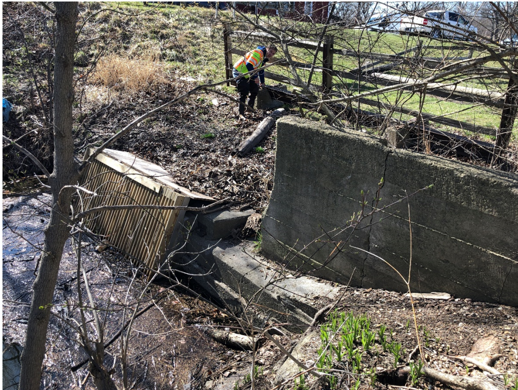
Figure 2: Existing millrace culvert inlet and headwall
