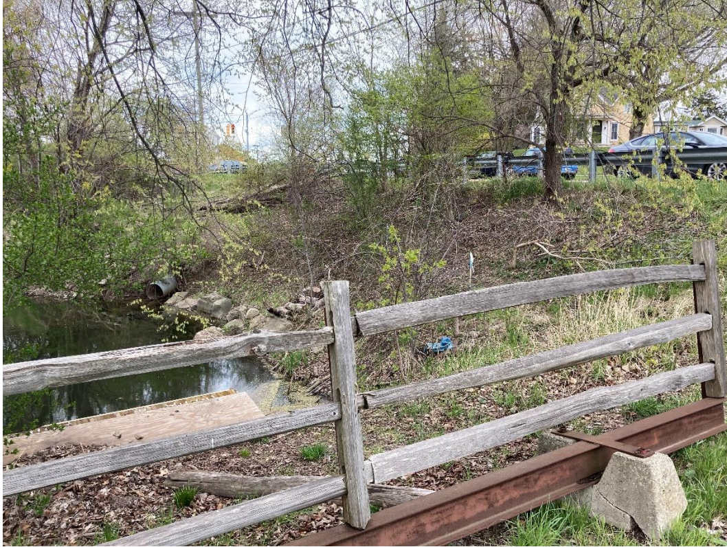
East Avon Road Lower Retaining Wall – Existing Site Photo Looking Northeast
