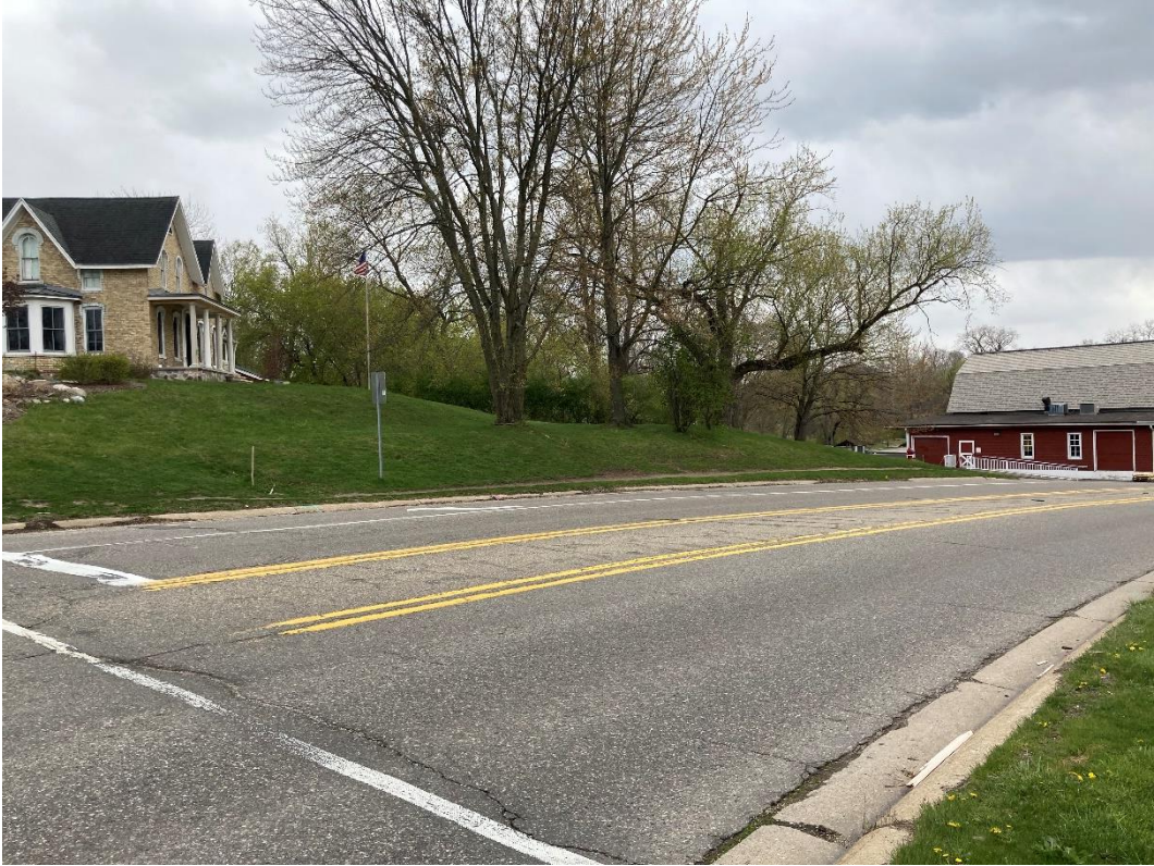
East Avon Road Upper Retaining Wall – Existing Site Photo Looking South
