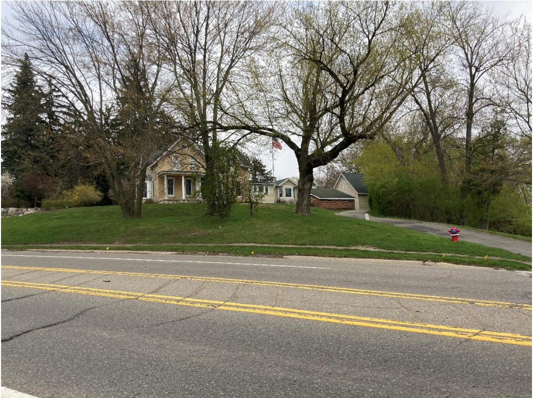
East Avon Road Upper Retaining Wall – Existing Site Photo Looking Southeast
