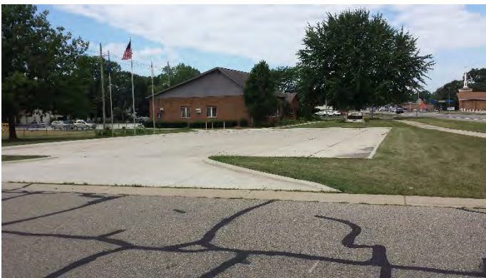
Looking west on the south leg of the intersection of Hessel and Auburn
