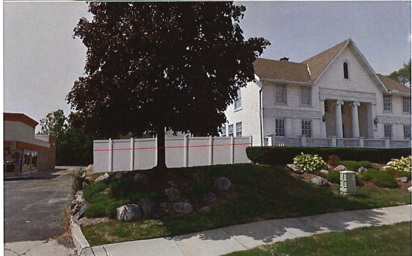
Red line indicates height of previous picket fence
