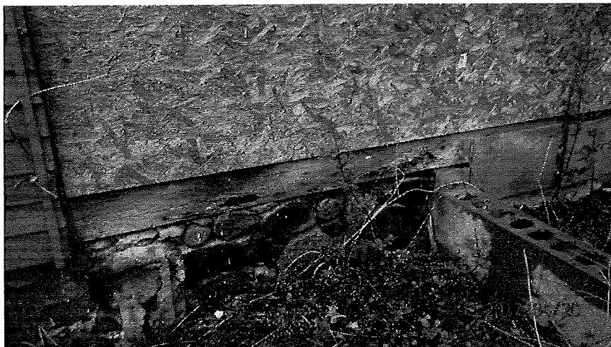
Sill and Foundation at South
