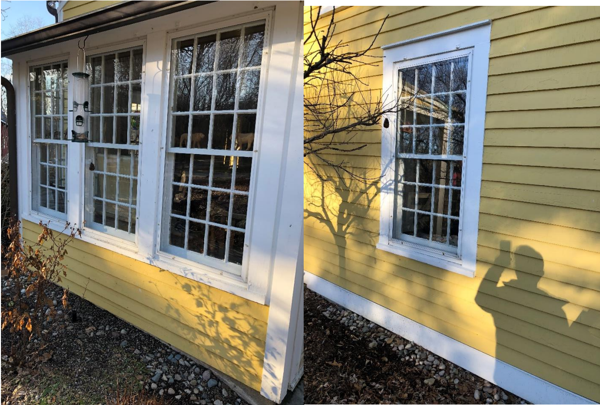
Photos of existing windows provided by applicant:
