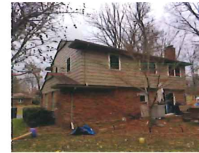
REAR ELEVATION - AREA OF ADDITION
