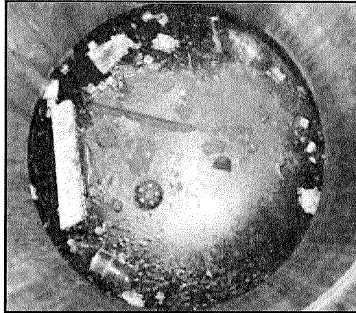
Floatable debris in the Aqua-Swirl®
