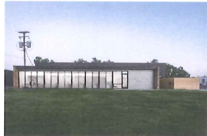
ONE CARE OFFICES - 2015 Troy, Michigan 17,000 SF "Commercial Design Office" 1st place, Detroit Home Design Awards, 2017
