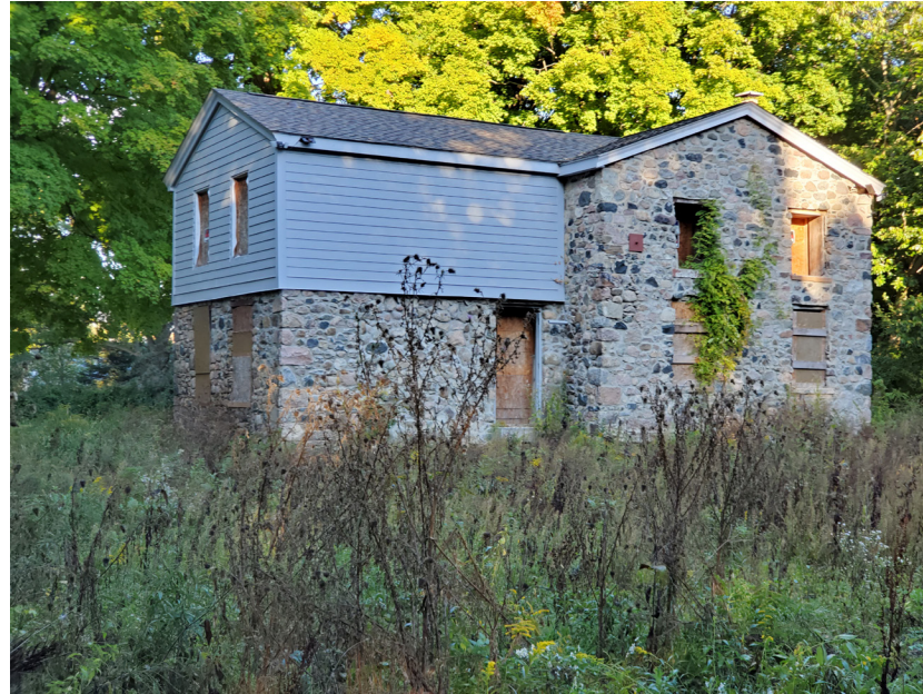
(A) LORNA STONE HOUSE - EXISTING VIEW FROM SE
