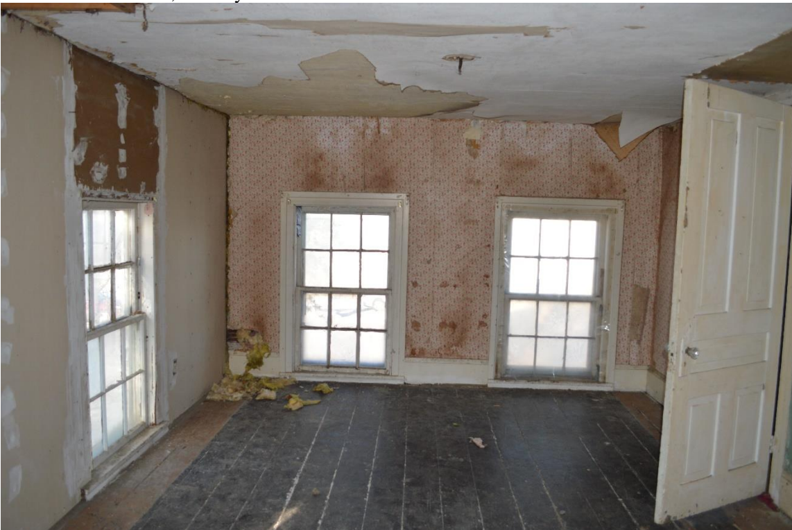
West room second floor, January 2015
