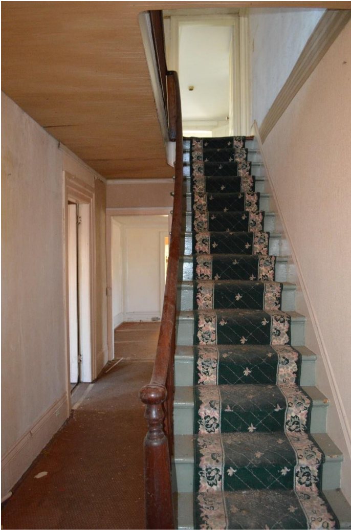
Central hall and stair, January 2015
