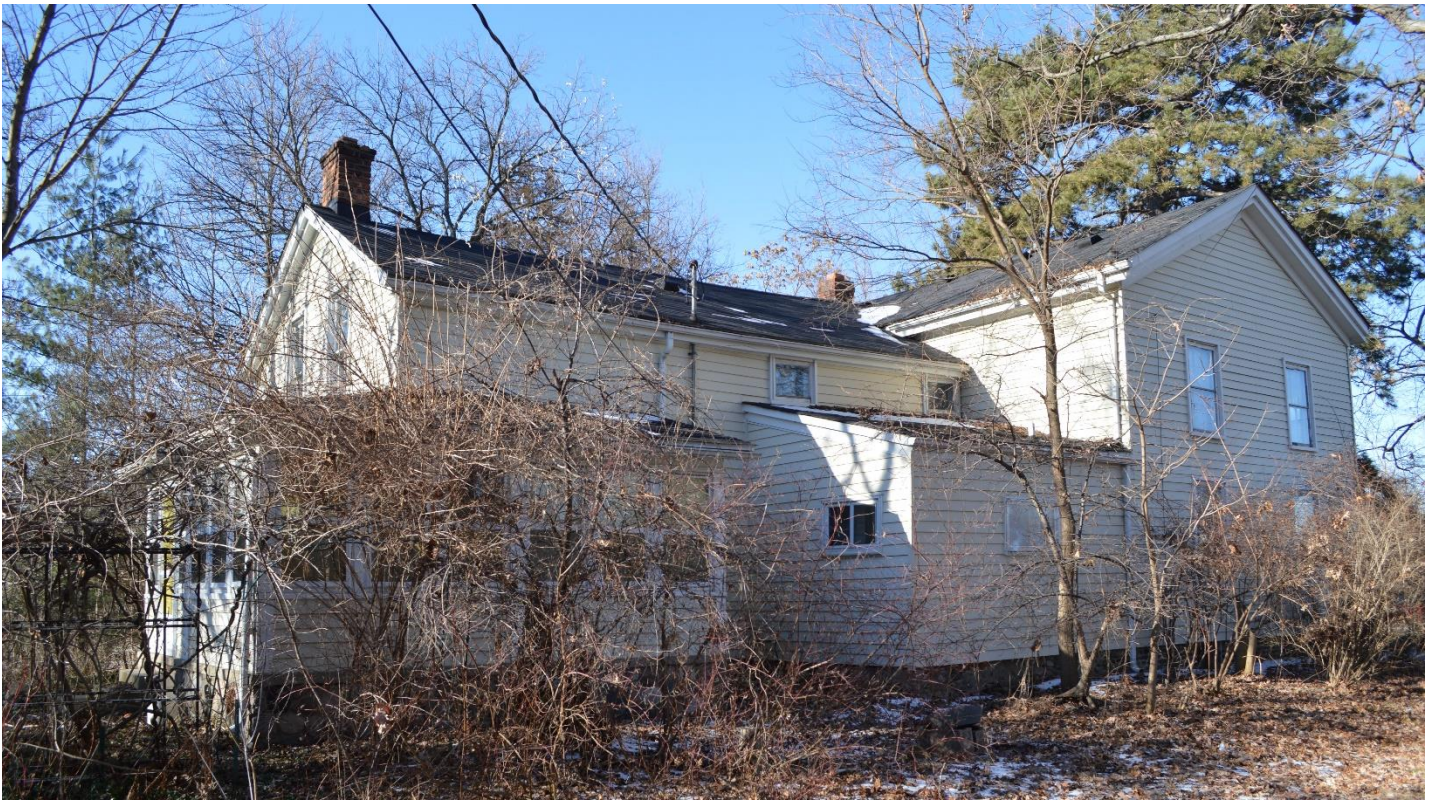
West and south elevations, January 2016
