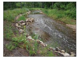
Examples of bank terracing (left) to repair a steep eroding bank, and vane arm (above) to redirect water back to the center of the channel
