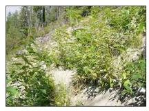
Steep slope stabilization in Canada, similar to conditions present at Cloverport. Severely steeped banks are cut back and terraced (left). Terraced landings are seeded and installed with live brush layers and wattles. Within several months, the slopes begin to vegetate (middle). Within 2 years, it is expected that the banks will be vegetated and stable (right).
