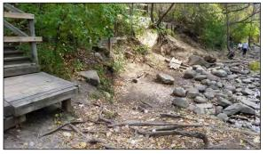
Significant bank erosion at the Yates Cider Mill property has led to portions of the trail being closed until restoration activities can repair the river
