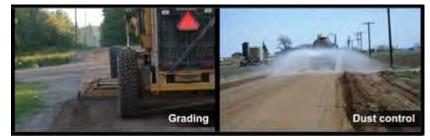
Figure 6: Examples of capital preventative maintenance treatments cont'd (left) gravel road undergoing maintenance grading, (right) gravel road receiving dust control application (dust control photo courtesy of Weld County, Colorado, weldgov.com)
