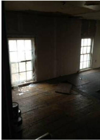
Windows set too closely to floor posing as safety hazards throughout second story of home.
