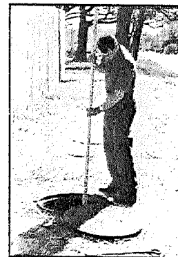
Sediment inspection using a stadia rod
