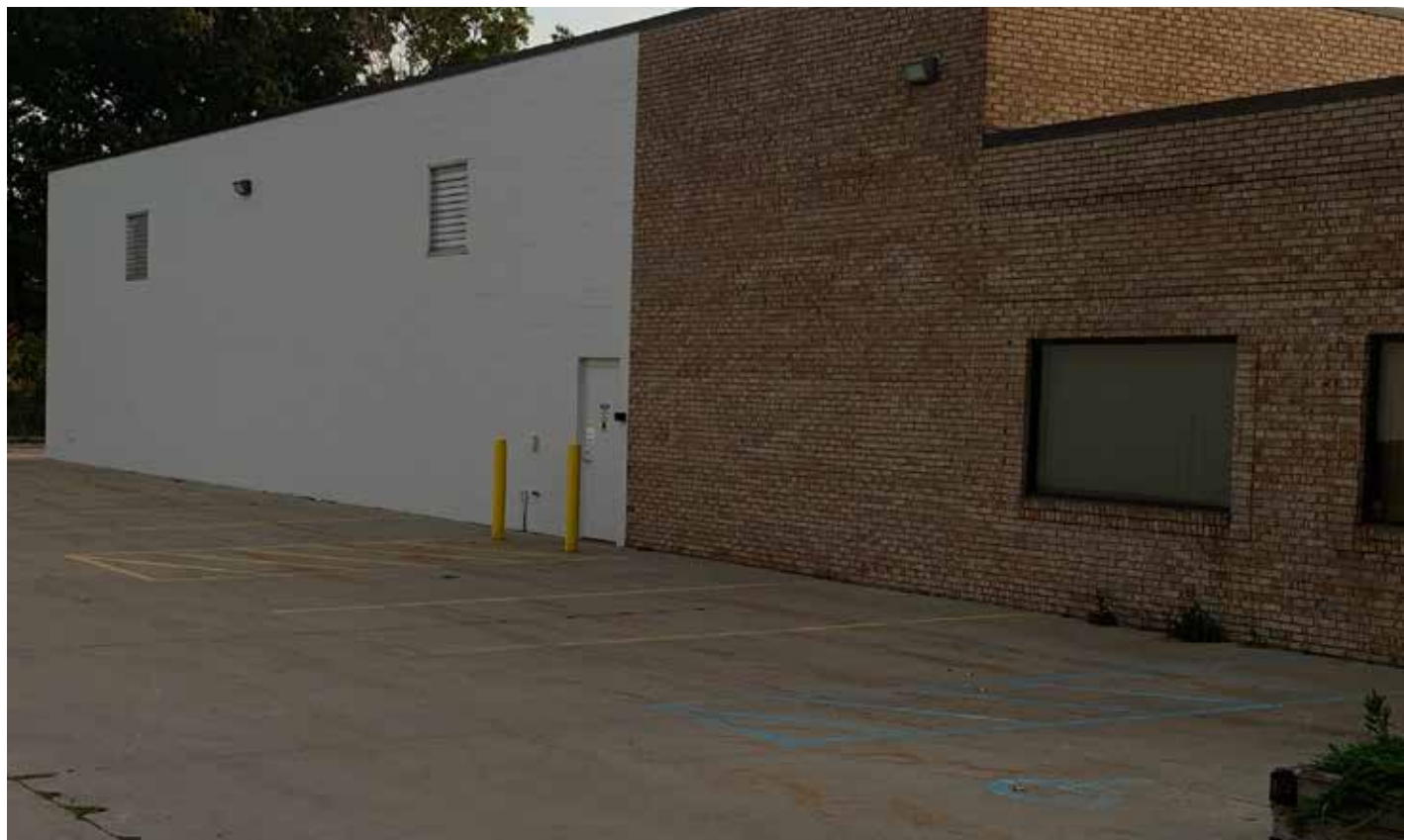
existing building - reference
