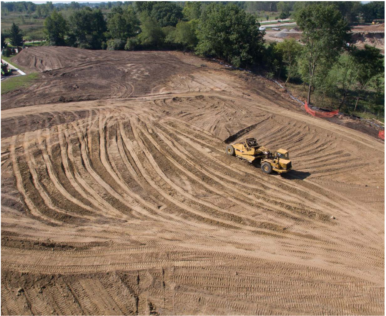
Park construction activities
